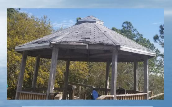
Wood was rotting due to missing shingles and leaking roof. Structural integrity was at risk without repair.
