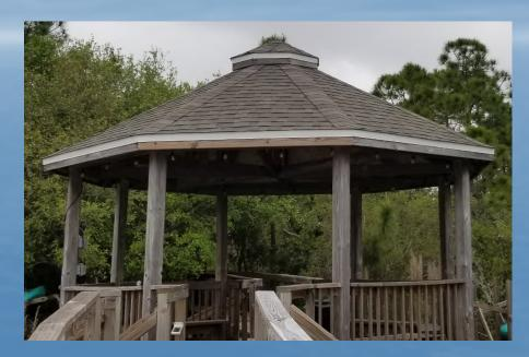
Old roof torn off. Roof decking boards repaired and replaced. Eaves boards replaced. Dimensional shingles installed.
